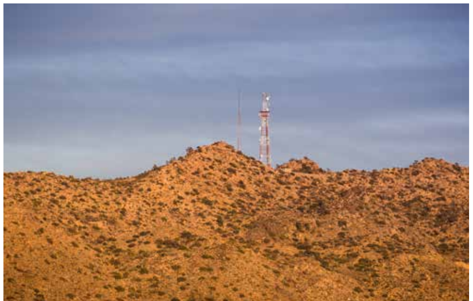
A telecom tower in California.
