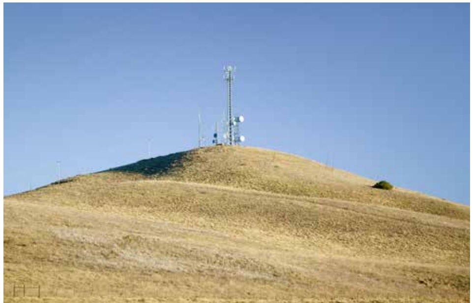
A telecom tower in California.
